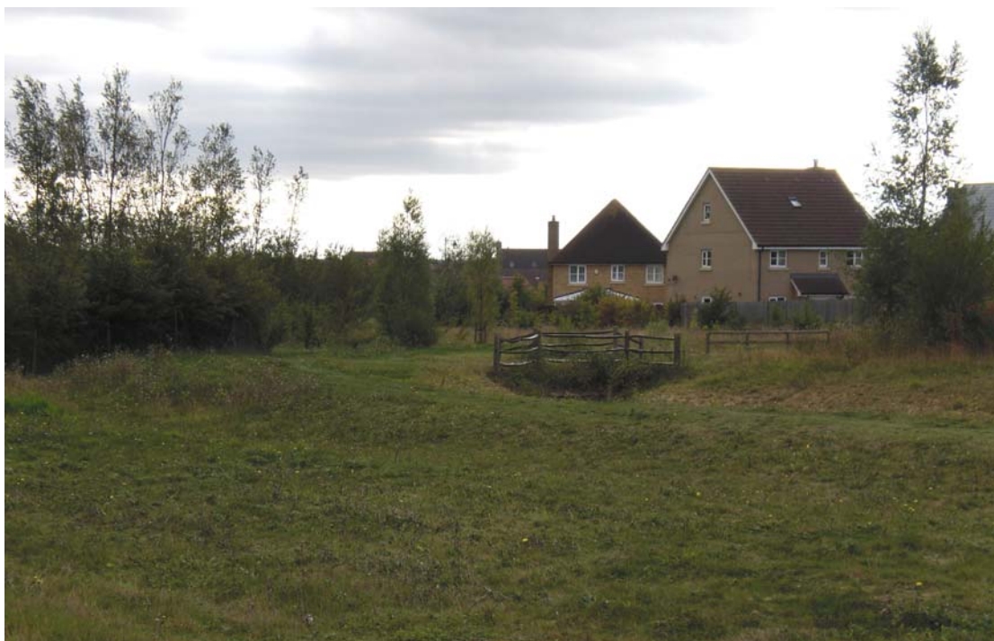
SUDS at Cambourne – Areas for water storage incorporated into public open space
